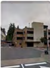
Standalone Parking Garage Near Businesses Bridgeport Village
