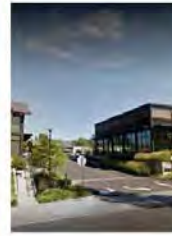
Internal Parking Surrounded by Buildings Kruse Village
